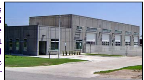
South elevation of the main building,
