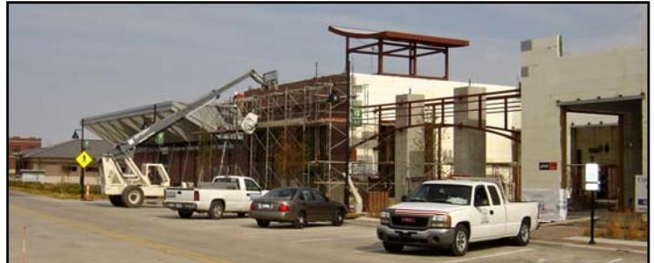
form (ICF) walls. At this time the ICF walls are complete, the steel will be finished by Dec. 1st and the masonry is progressing well. Architect for this project is Matt Cortez of GLMV Architecture. The Estimator/Project Manager is Gib Compton. David Spoon is the Job Superintendent. The building is scheduled to be completed in May.
